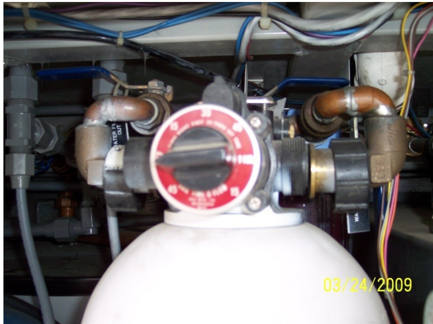
Water Line Connections “ Top of Filter”
