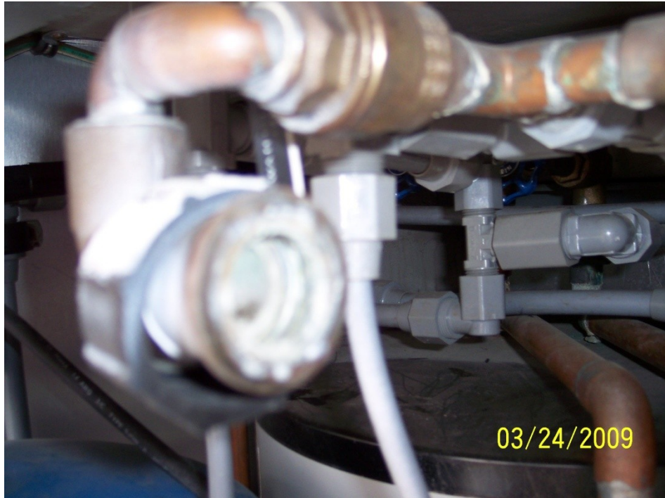
Outlet Line with Sand Filter Removed
