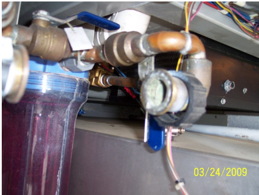
Inlet Line with Sand Filter Removed
