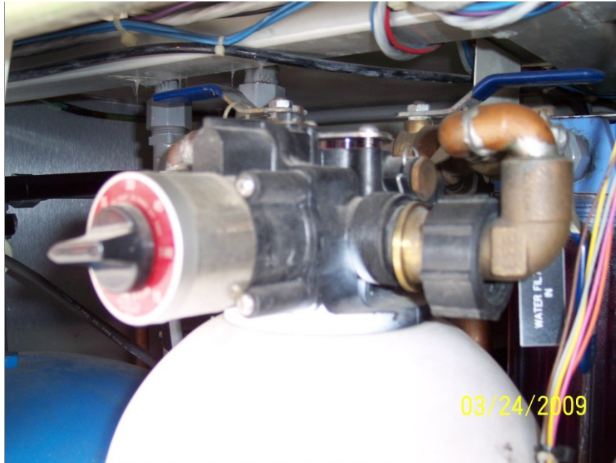
Right Hand or Forward " INLET SUPPLY LINE " Connection / Coupling
